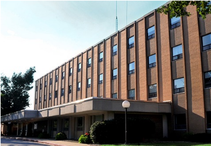
The exterior of St. Francis Hospital. Photo courtesy of St. Francis Hospital website .
